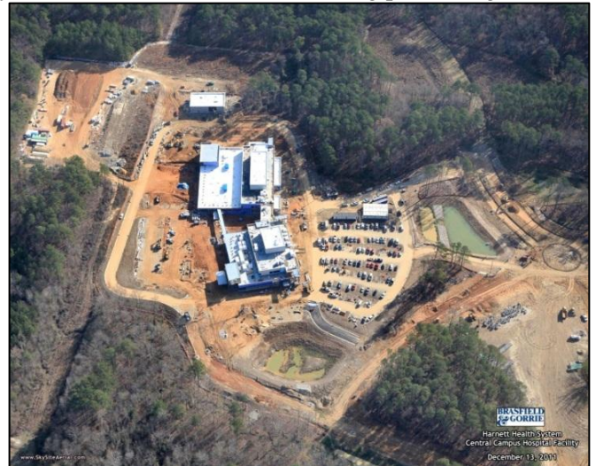
December aerial photo, HHS Facility
